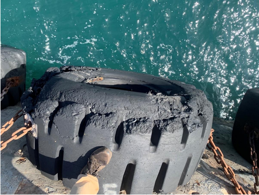
Photo 3: Example of the five (5) tire fenders to be replaced along with chains and new shackles.
