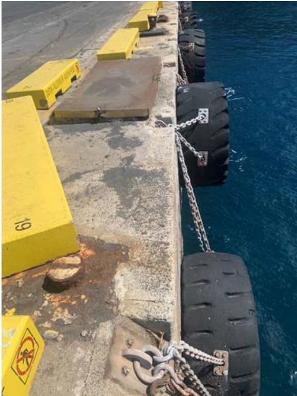
Photo 1: Existing Tire Fender system to remain
