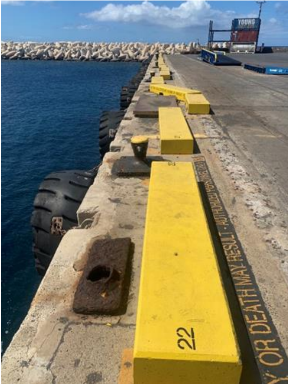
Photo 2: View of existing pier.
